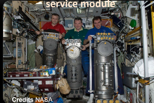
Elektron units in the Zvezda service module
